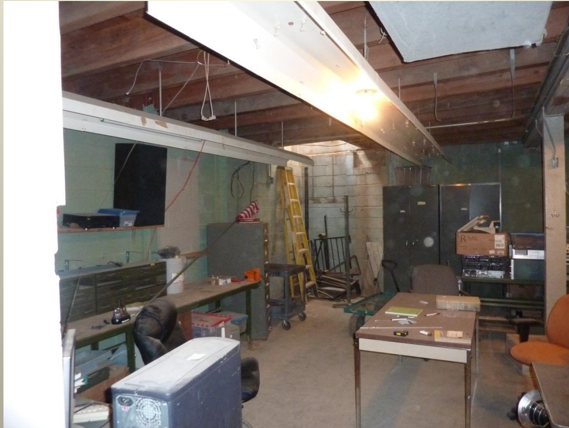
Main bunker room looking west.
