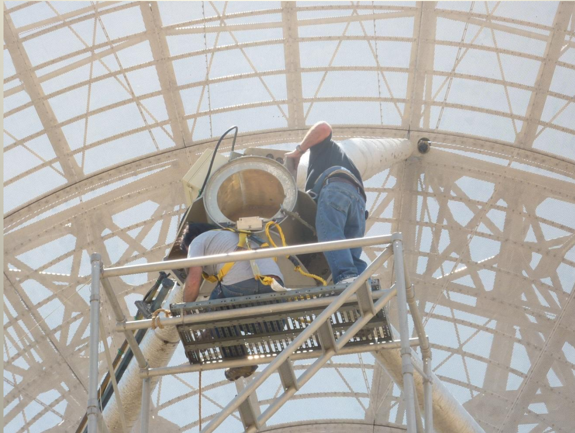
Install of 1296 Mhz antenna feed
