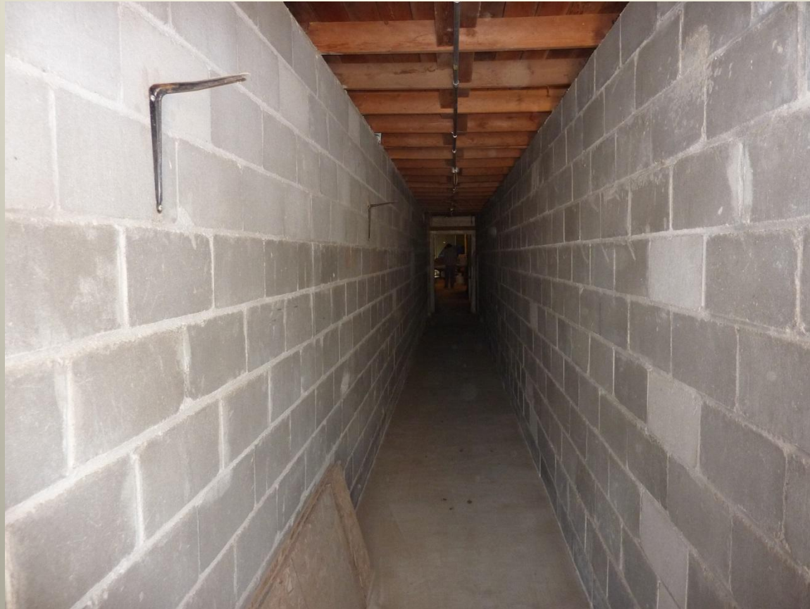
Looking from bunker entrance to main bunker rooms
